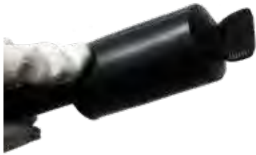
1. Slide the HSIC-FR end cap onto the cable and hold in place using forefinger or thumb.
